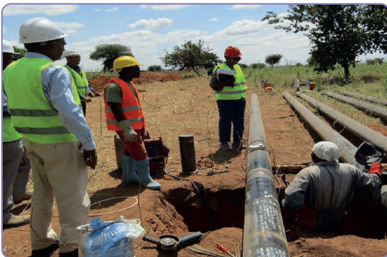
Workers at Majohe Water Project site, Dar es Salaam
